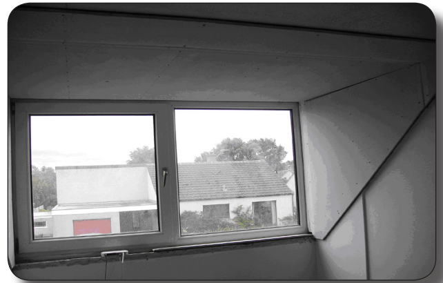
Spacetherm Fermacell Panels installed on the combed dorma
