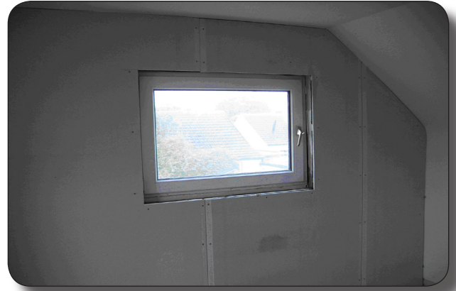
Spacetherm Fermacell Panels installed on the gable end
