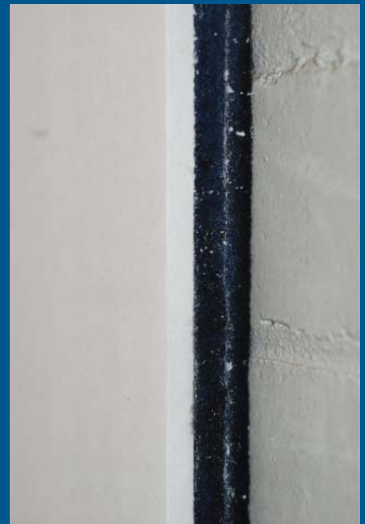
Close up view of Spacetherm after installation
